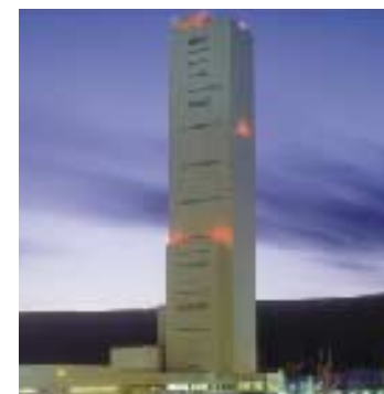
Bristol Test Tower, USA
