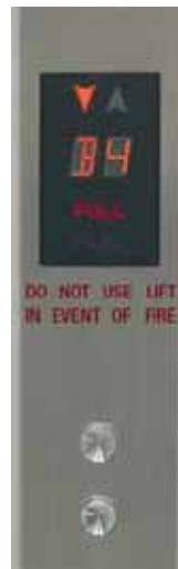
Combined Hall Button and Hall Position Indicator
